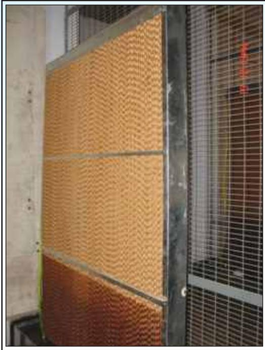
Fan - pad system fitted at poultry shelter, Poultry Farm, Department of Livestock Production Management, COVS,GADVASU
